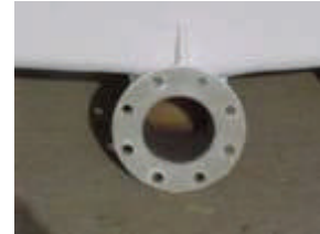
Flange on sump
